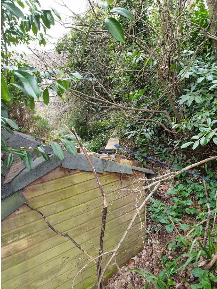
Retaining wall running across north/Westcote Road side of site
